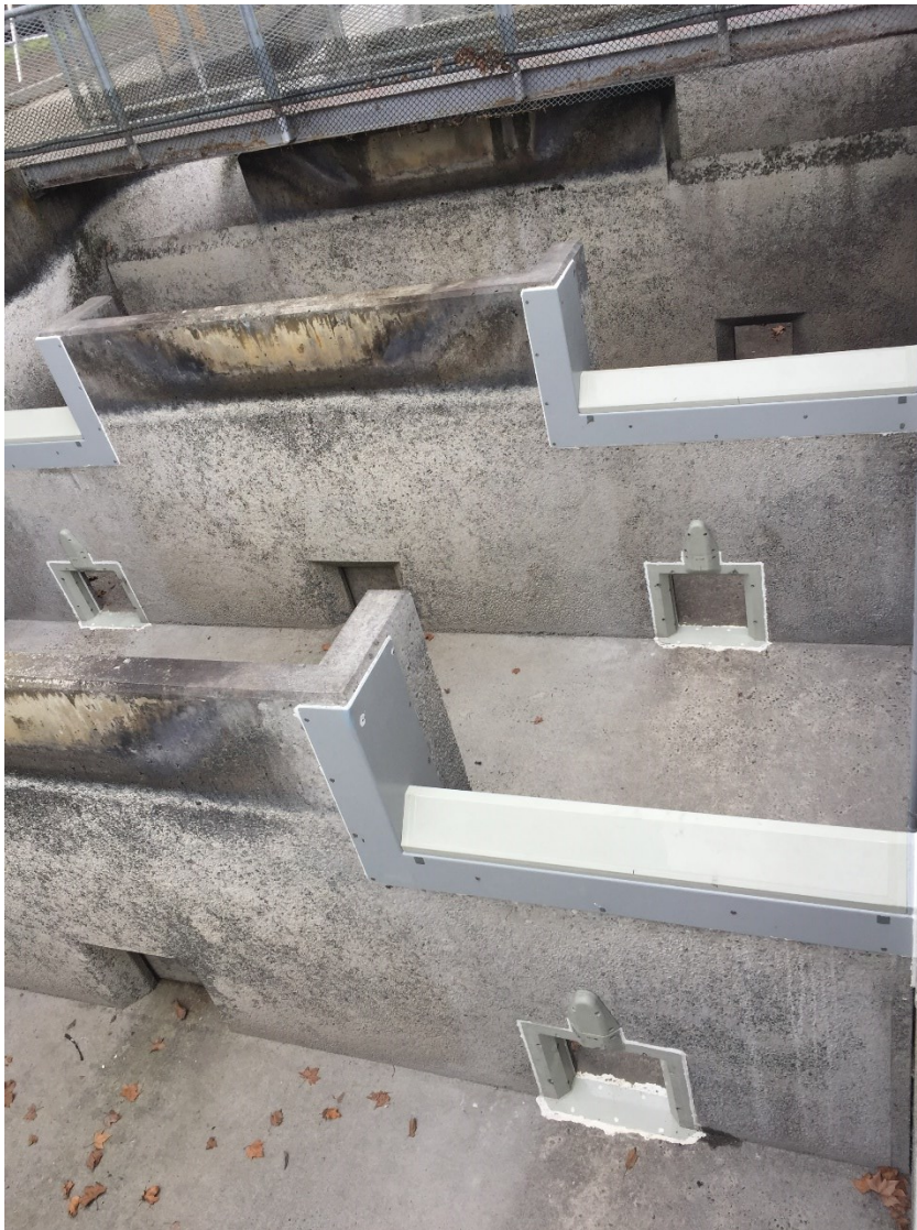
Figure 8. John Day Dam adult ladder orifice and overflow antennas.
